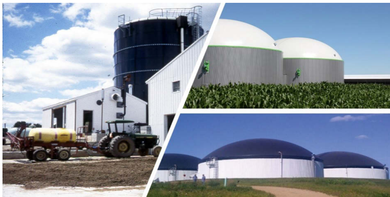
Figure 3.11. Examples of Complete Mix Digesters 29
