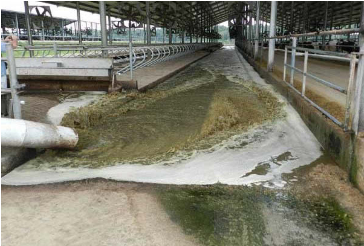
Figure 4.4. Dairy Manure Alleyway Flushing 36
